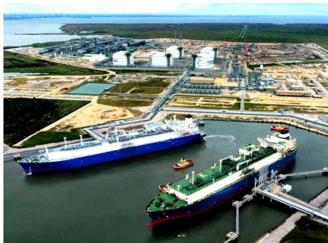
Sabine Pass LNG Export Terminal, Cameron Parish, Louisiana (Photo courtesy of Cheniere Energy, Inc.)
